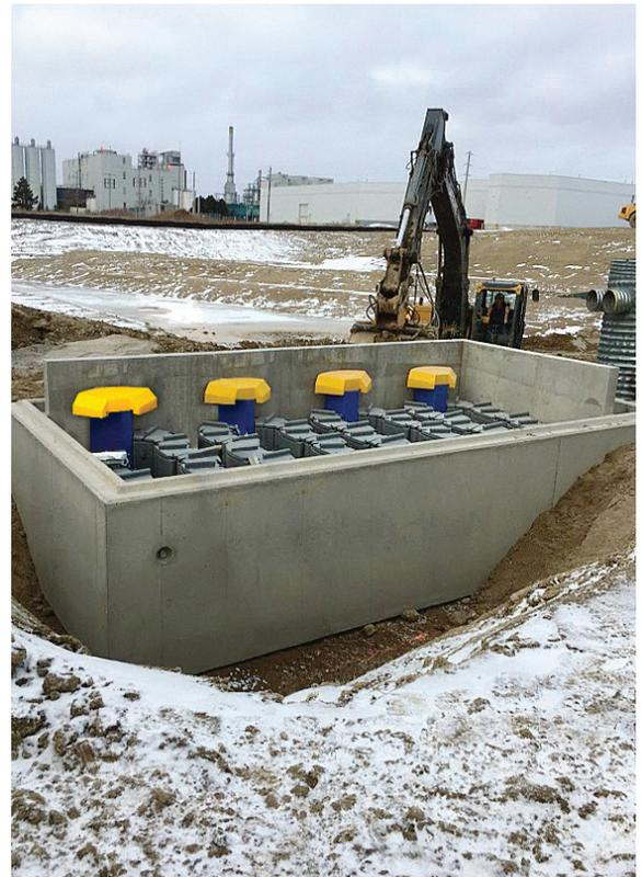
The system is certified by the New Jersey Department of Environmental Protection (NJDEP) and the City of Toronto, to have a removal rate of >80% Total Suspended Solids (TSS). This was critical to the project as the water would eventually flow into the existing storm sewer network.
