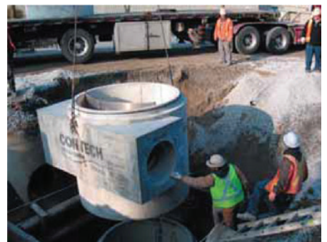
York Region sewer upgrade.
