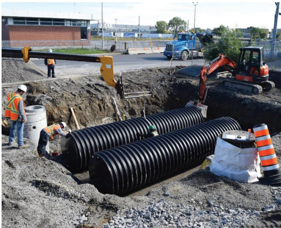
With a very narrow product specification in hand, the contractor on the project, Construction Arcade, quickly learned that there was a single solution that would meet all of the City's requirements - including the corrosion-resistance to gases and acids present in sanitary sewer systems.
